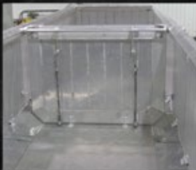
Walkthrough Center Gate/Baffle
